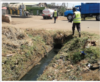
A well-maintained side drain
