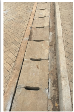
A well-maintained culverts
