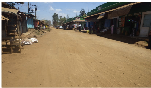
Repaired by patching the potholes
