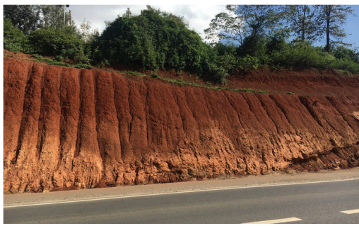
A well-maintained slope.
