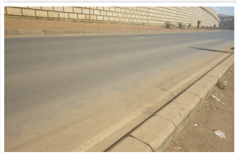
A smooth carriageway without crack
