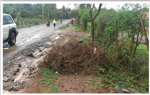
Unpaved footpath with obstruction
