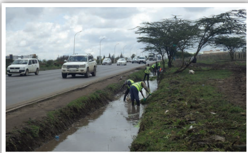
A well-maintained side drains
