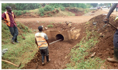
✅ Workers de-silting inlets/outlets of a culvert using a long handle shovel
