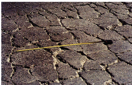
❌ Typical cracking
