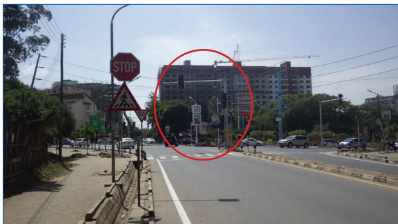
5. Traffic signal : Signal not facing traffic directly
