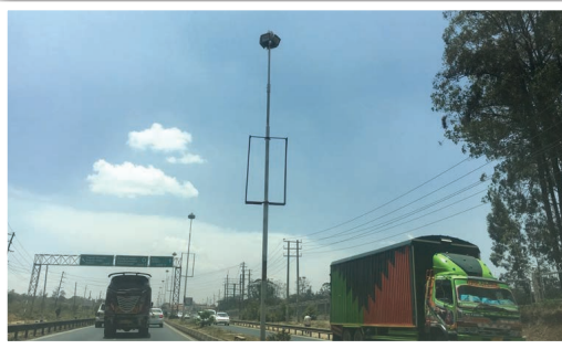
A carriageway with street lights
