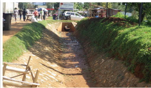
A well-maintained condition
