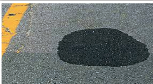
✅ Repaired by patching the potholes
