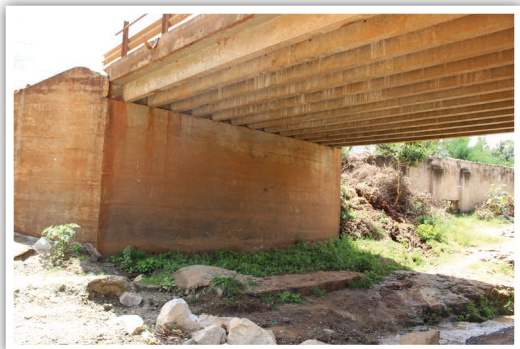
A proper bridge abutment
