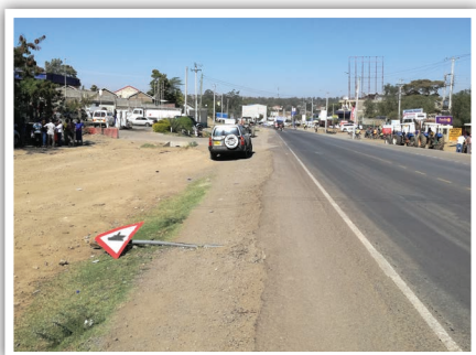
The traffic signal knocked down
