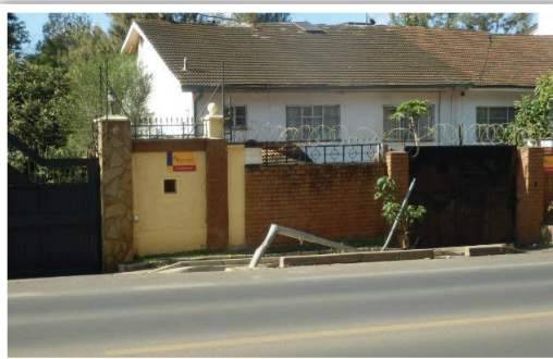
Damaged street lights
