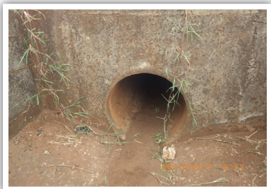
✅ A well-maintained cross culvert
