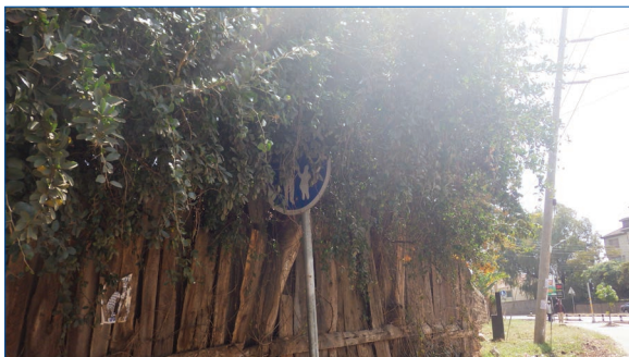
6. Vegetation obstructs visibility
