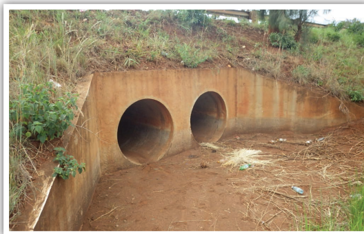
✅ A well maintained box culvert (case of pipe culvert)
