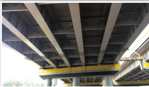
The steel structure is in good condition
