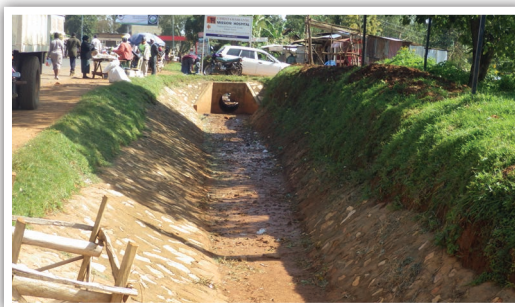
Well-maintained side drains along the road
