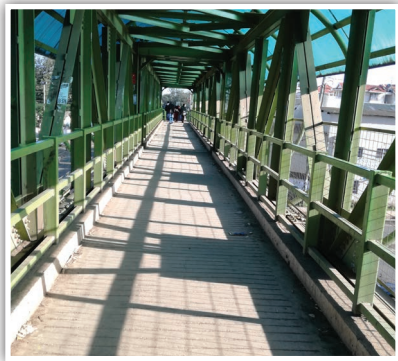
The steel structure is in good condition.
