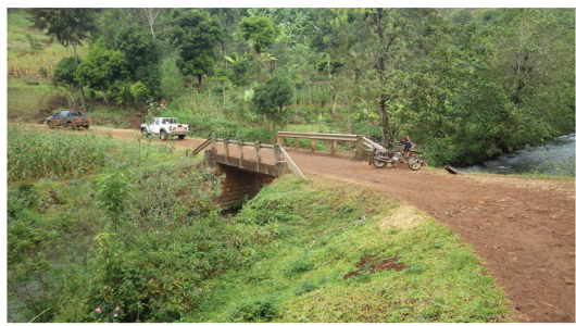
The bridge is working well
