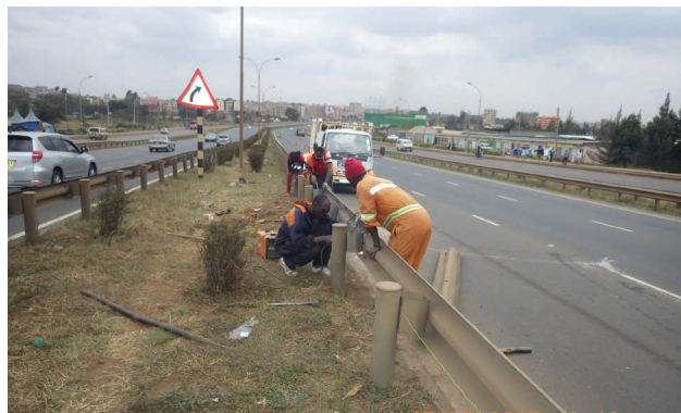
Fixing of straightened beam
