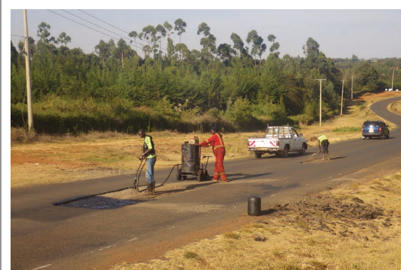
Spraying of Tack Coat
