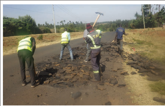
Removal of Cut Asphalt
