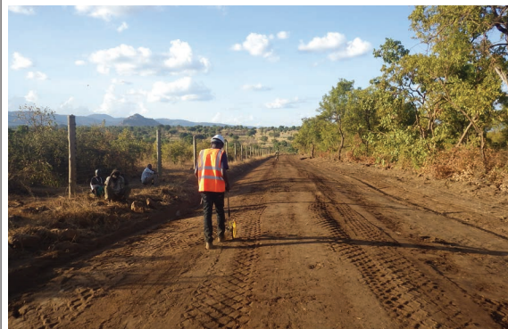
Measurement of Graded Area
