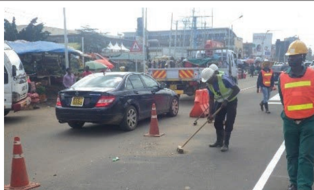
Cleaning of Road Surface
